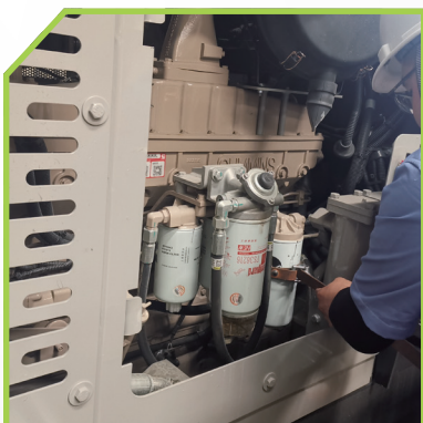
Oil filter maintenance
