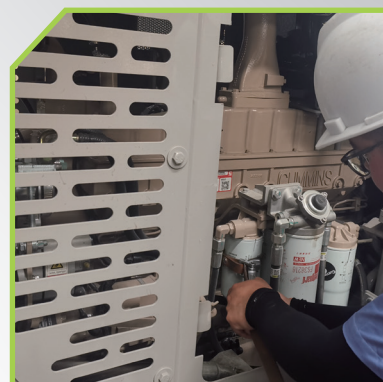
Fuel filter maintenance
