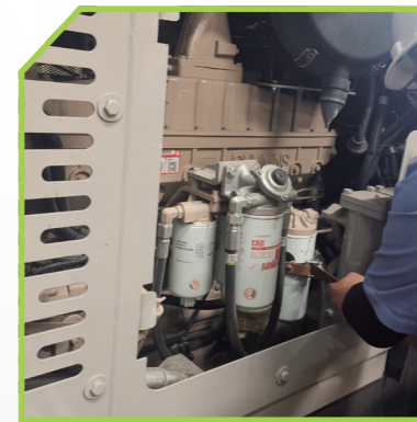
Oil filter maintenance 机油滤更换
