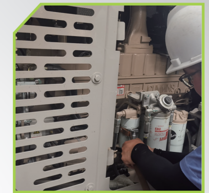
Fuel filter maintenance 燃油滤更换
