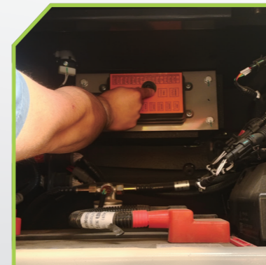
Replacing fuse 保险更换
